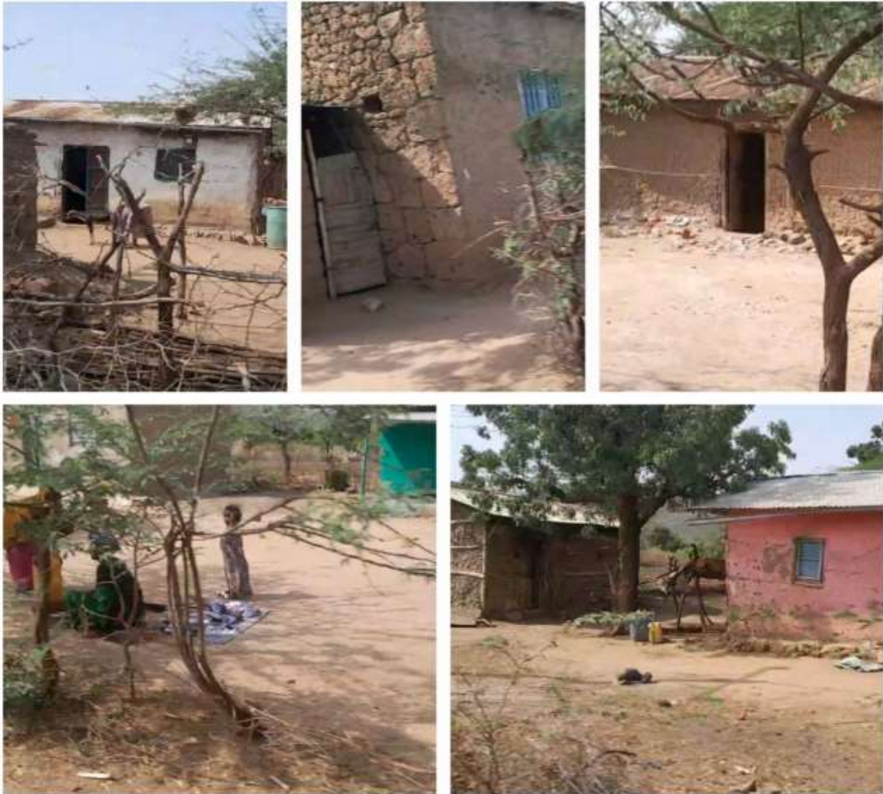
Figure: Scattered individual residential properties at Hula Hulul kebele
